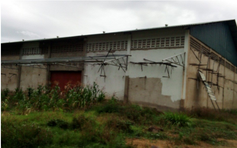
A4.2 Scheme's warehouse in Mkula village
