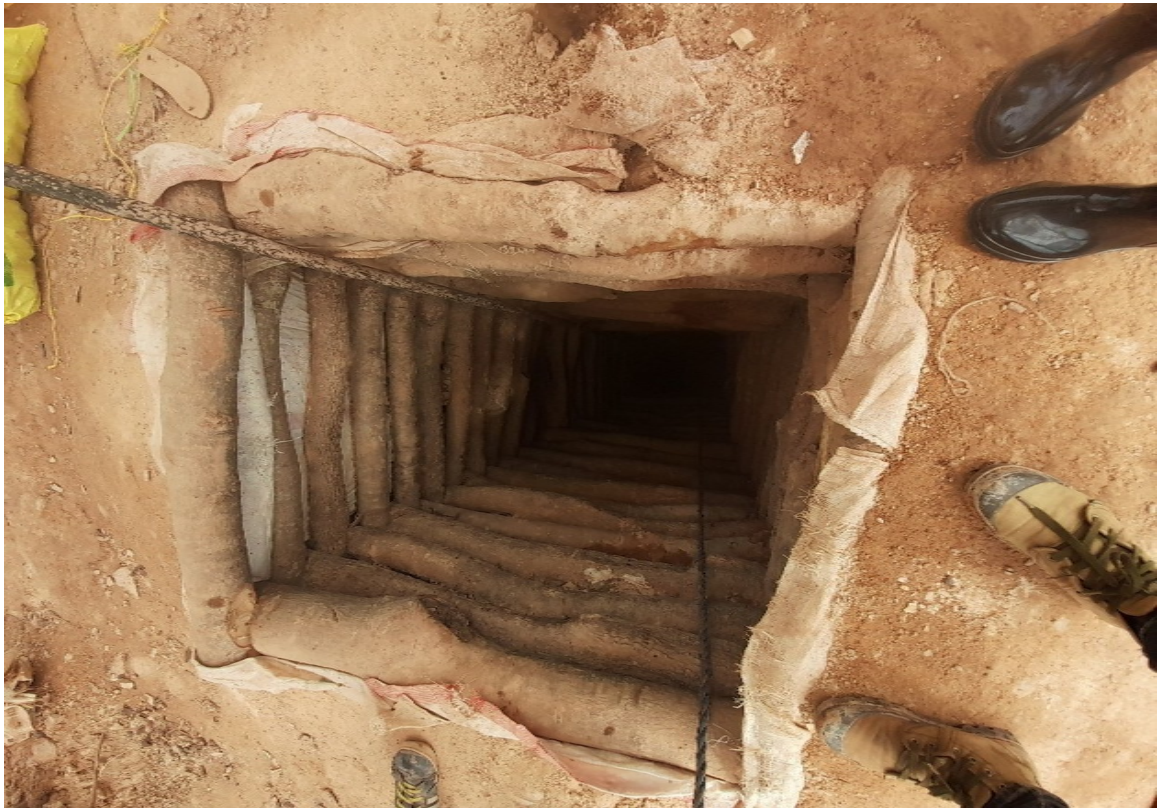
Plate 3.1: Pit constructed using Brachystegia spiciformis .
