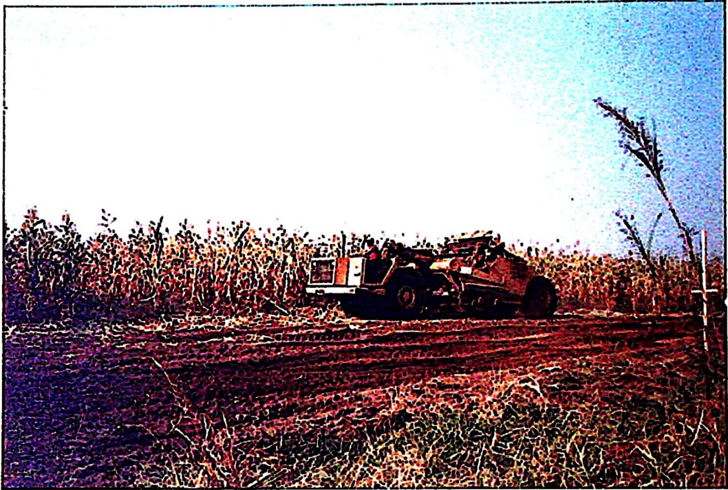
Figure 5.6. Construction of the embankment of grassed waterway A
