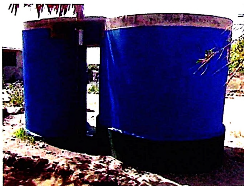
Fig. 7. 1. A community-scale defluoridation plant at a village school (Dahi, 2016)
