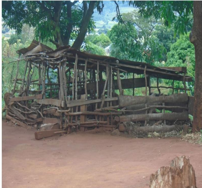
Fig. 2 Pigpen construction with clay floor and wood fence
