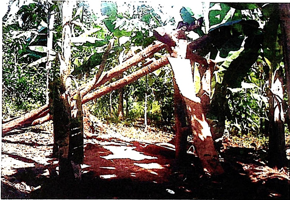
Plate 1: Platform construction (Photo by Kway, 1997)
