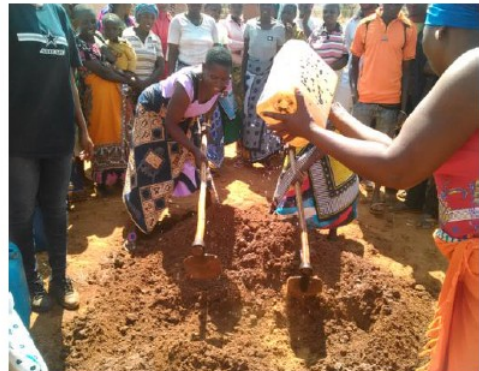
4. Mix soil, manure, sand and water.
