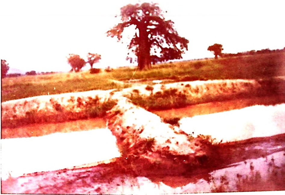
Plate 4.5: Storage reservoir full of runoff (March 1995).
