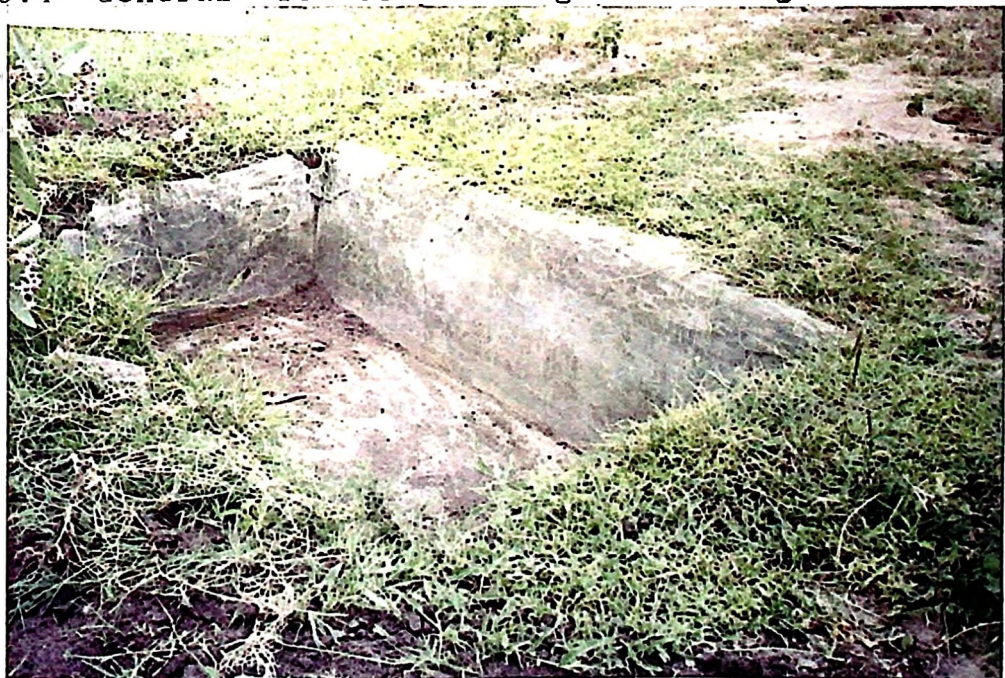
FIGURE 3.5 General view of Excavated collecting tank.
